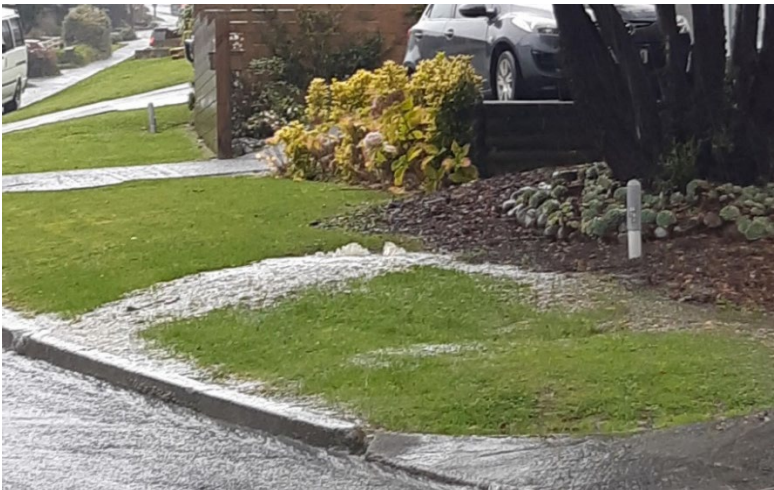
Figure 2-4: View of an uncontrolled overflow from a manhole into a nearby kerb and channel
